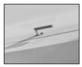
The manual Neo® is operated with a satin finished handle. The handle is pre-installed at the cill of the roof window. To open, turn the handle clockwise and lift; it will remain open with the support of the gas springs. To lock the window, carefully lower the casement and when closed, turn the handle counter-clockwise. For out of reach Neo® roof windows a pole winder can be used (see manually operated ironmongery above).
